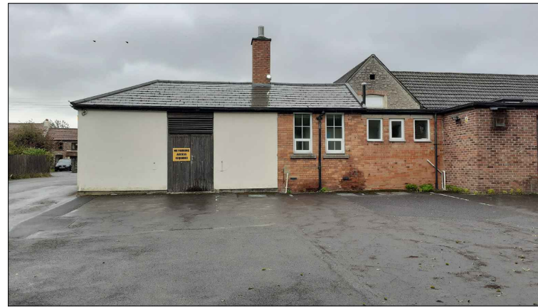
View of boiler room and toilets
